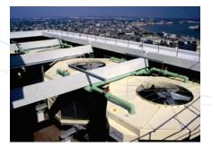
Marley QuadraFlow<sup>®</sup> Cooling Tower— Induced-draft, low profile design. These fiberglass and stainless steel towers are field assembled to facilitate siting, and are available from 129 to 1,047 tons per cell. CTI Certified.
